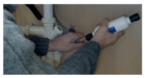
The filter has a flow arrow pointing in the direction of the water flow. This indicated where the "in" and "out" goes, so ensure you have the filter pointing in the right direction for your water flow. Your filter comes with a mounting clip which you can position accordingly.
