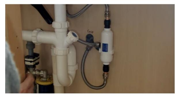
Once the filter is in position, you can turn on the cold water supply and check for any leaks.Run the filter for at least 5 minutes to flush the filter of any loose carbon or sediments.
