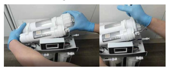
Insert the membrane into the membrane housing. Ensure it goes into the socket at the other end of the housing inside it and the membrane is flush with the top of the housing.
