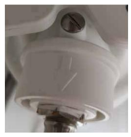
FIG3: DIRECTIONAL ARROW OF WATER FLOW
