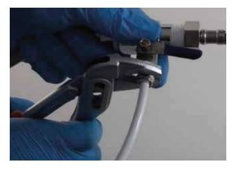
The Feed in valve connects to the cold hose of the existing cold tap on the sink.
