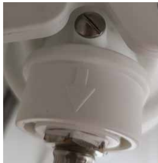
FIG3: DIRECTIONAL ARROW OF WATER FLOW
